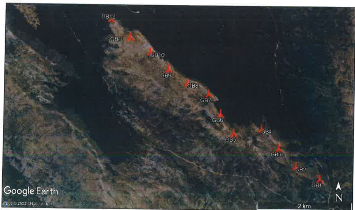
Figure 1 Wind Farm "Bundina kosa" area with Wind Turbines
